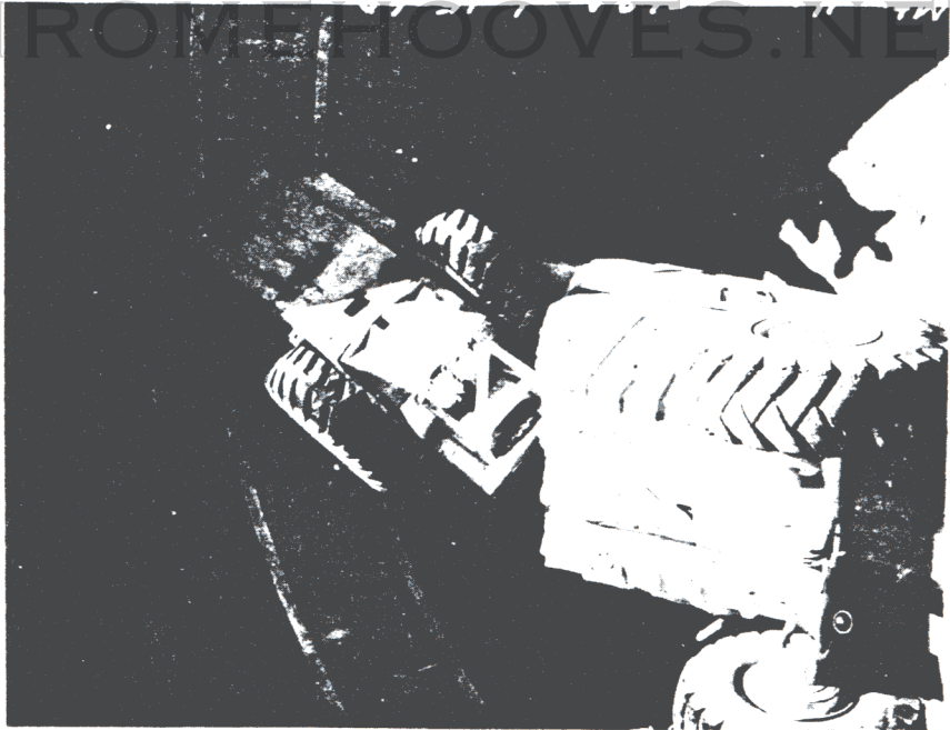
Fig I 15 June 1960 Complex 1A Propellant Terminal No. 2 - Position of "C" Pull After Backing into Propellant Terminal
