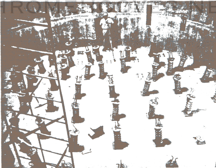
Fig I 2 September 1960 Complex 1C Propellant Terminal - Coil Spring Mounts
