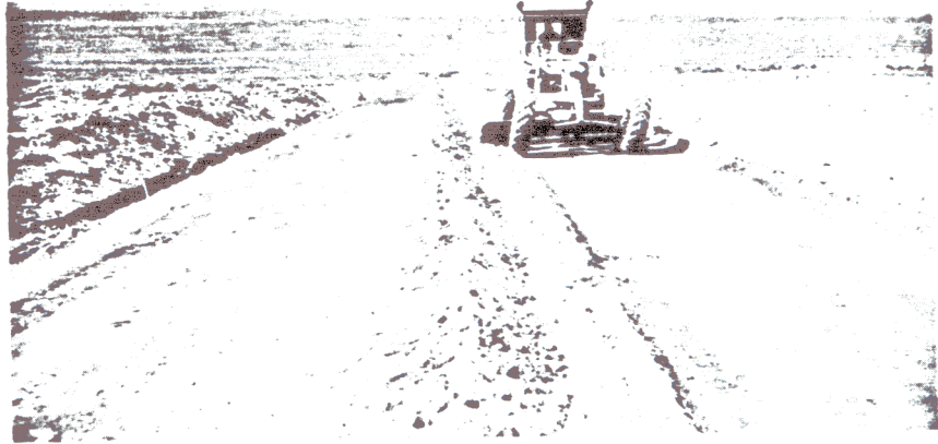
Fig I 22 March 1960 Complex 1A Access Road Construction - Looking Toward Hiway 51
