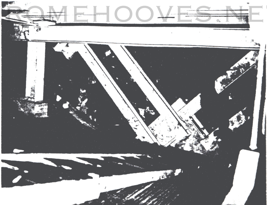
Fig I 15 February 1962 Complex 1A Portal Silo - Painter, Fatal Fall Spring Beams Indicate Body Position
