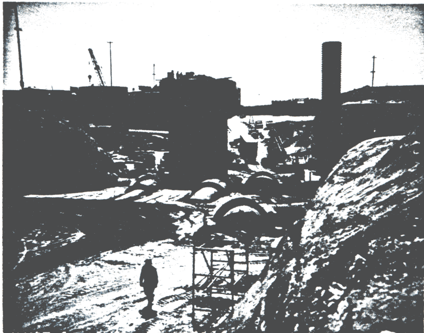
Fig II 28 April 1961 Complex 1C Powerhouse Area - Backfill
