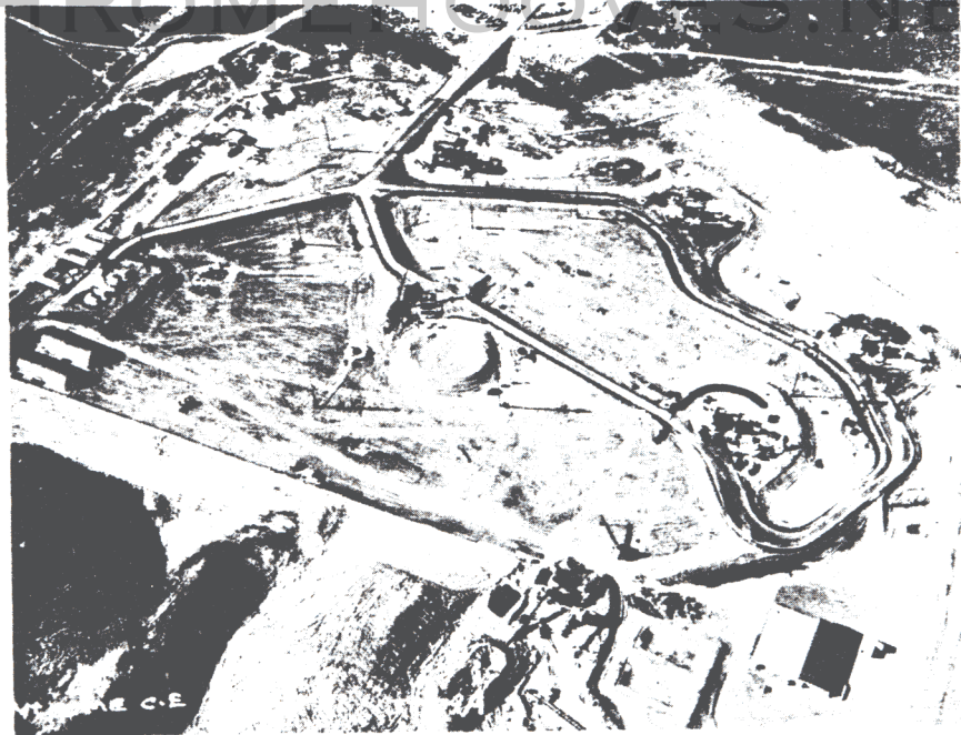
Fig I 31 October 1961 Complex 1A Over-All View - Looking Southwest
