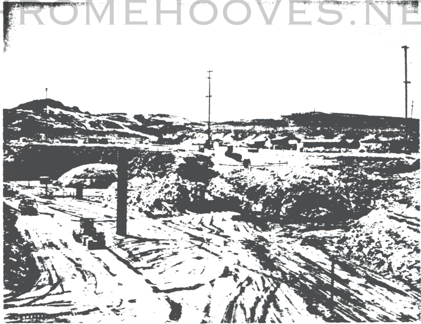
Fig I 12 July 1961 Complex 1A Blast Lock No. 2 Area - Backfill
