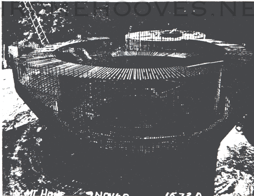
Fig I 9 November 1960 Complex 1A Missile Silo - Reinforcing Steel
