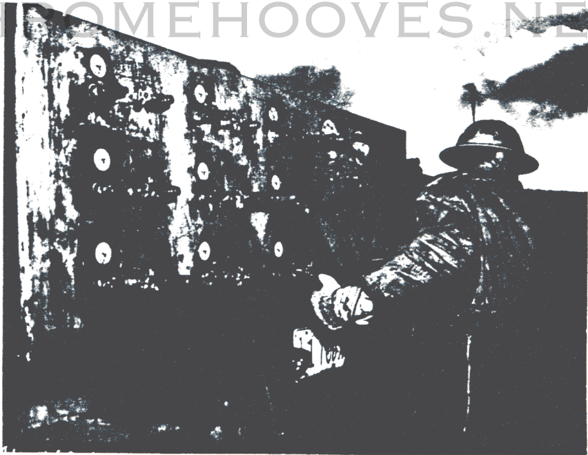
Fig I 21 December 1960 Complex 1A Central Pneumatic System for Multiple Jacking
