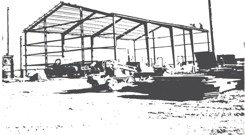
Fig I 7 February 1961 Liquid Oxygen Plant - Steel Framing Complete
