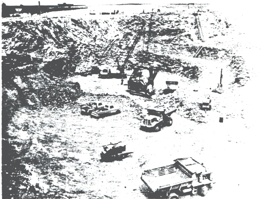
Fig II 24 May 1960 Complex 1A Powerhouse Area - Mass Excavation
