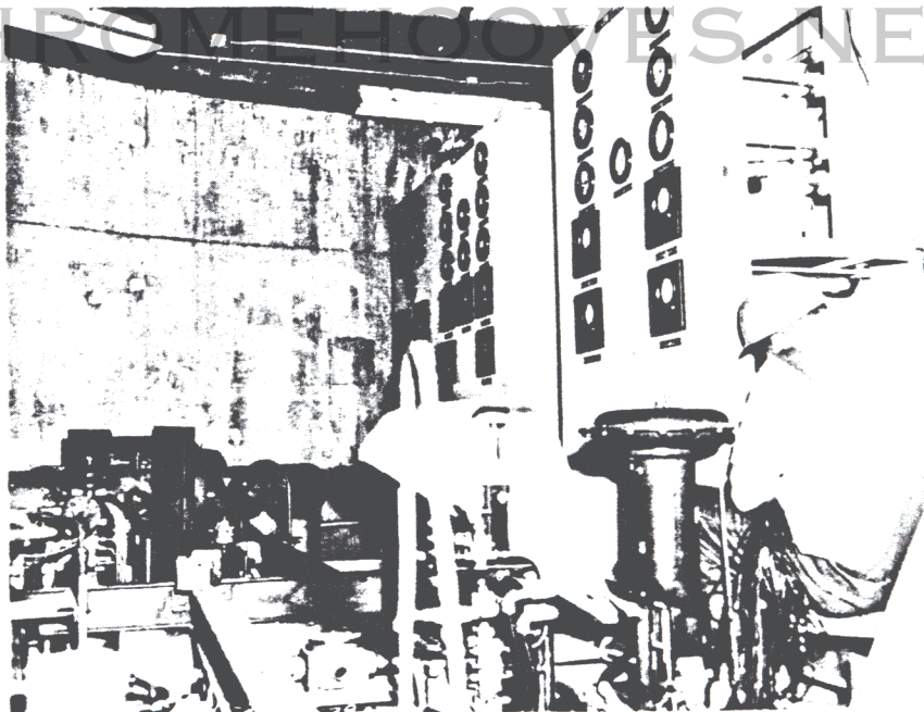
Fig I 29 November 1961 Complex 1B Propellant Terminal - LOX, Helium and Nitrogen Transfer Panels
