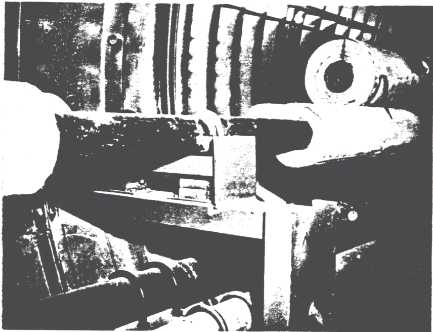
Fig II 9 February 1962 Complex 1A Equipment Terminal No. 2 - Pipe Supports in "A" Tunnel
