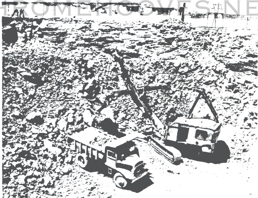
Fig I 1 June 1960 Complex 1A Antenna Silos - Mass Excavation
