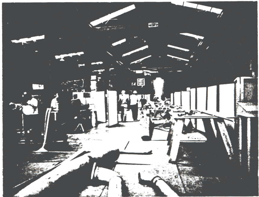
Fig II 14 June 1961 Grafe-Weeks Plant Subcontractor's Pipe Fabrication Shop
