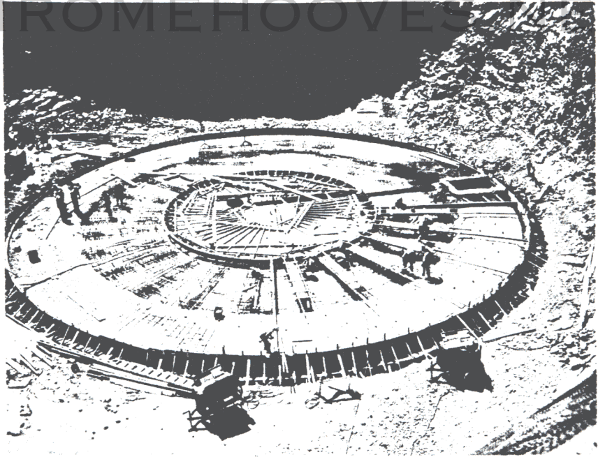
Fig I 19 July 1960 Complex 1A Control Center - Floor Form Preparation
