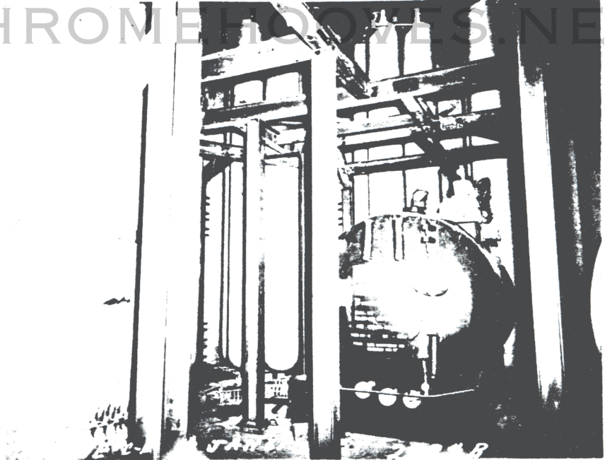
Fig I 19 January 1961 Complex 1B Propellant Terminal - Helium Cooler, T-402, Surrounded by Gaseous Storage Vessels
