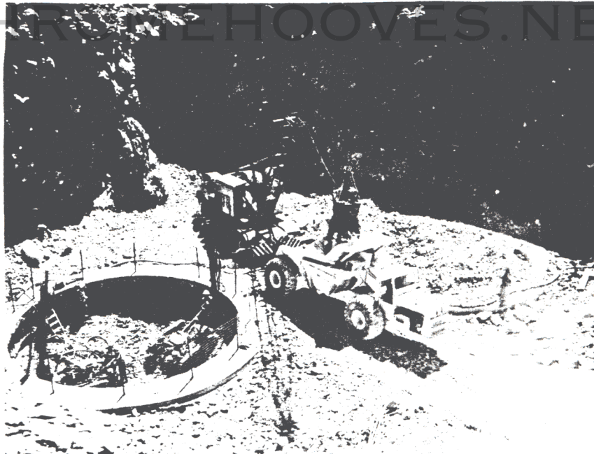
Fig I 3 August 1960 Complex 1A Air-Trac Drilling and Antenna Silo Excavation
