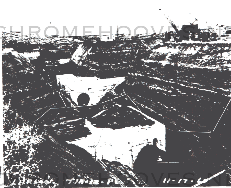
Complex 1-A - View Looking North at Blast Locks No. 1 and No. 2 and Interconnecting Personnel Tunnels. (Figure 23)
