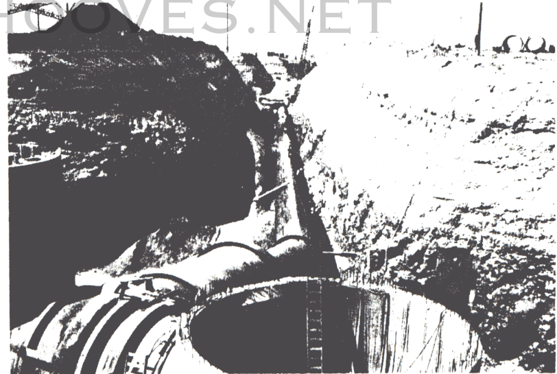
Personnel tunnel from antenna silos showing terminal junction in place and typical cut sections
