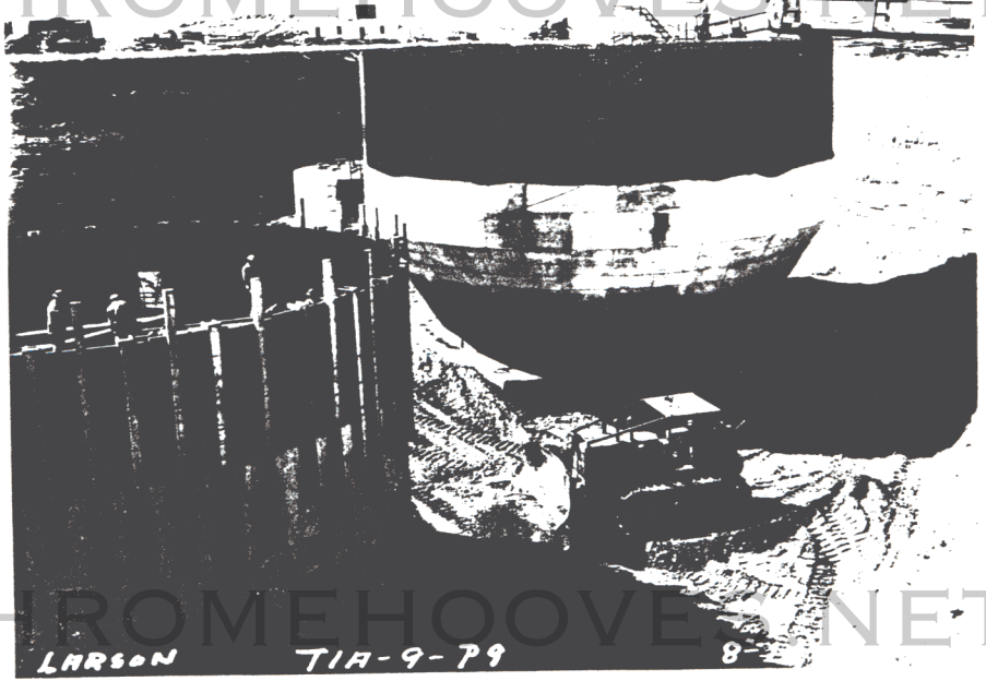
Complex 1-A view of Top of Missile Silo (Center) after Stripping Forms for Concrete Pour II, Pour 12 Will Cover Exposed Reinforcing Steel - Aug 61. (Figure 19)
