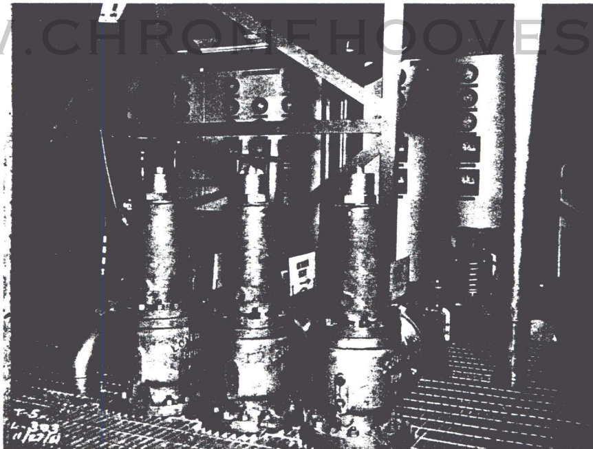
Fig. 92 Propellant Terminal, Main Deck (Completed installation of LOX tank safety valve manifold)(Transfer panels in background)
